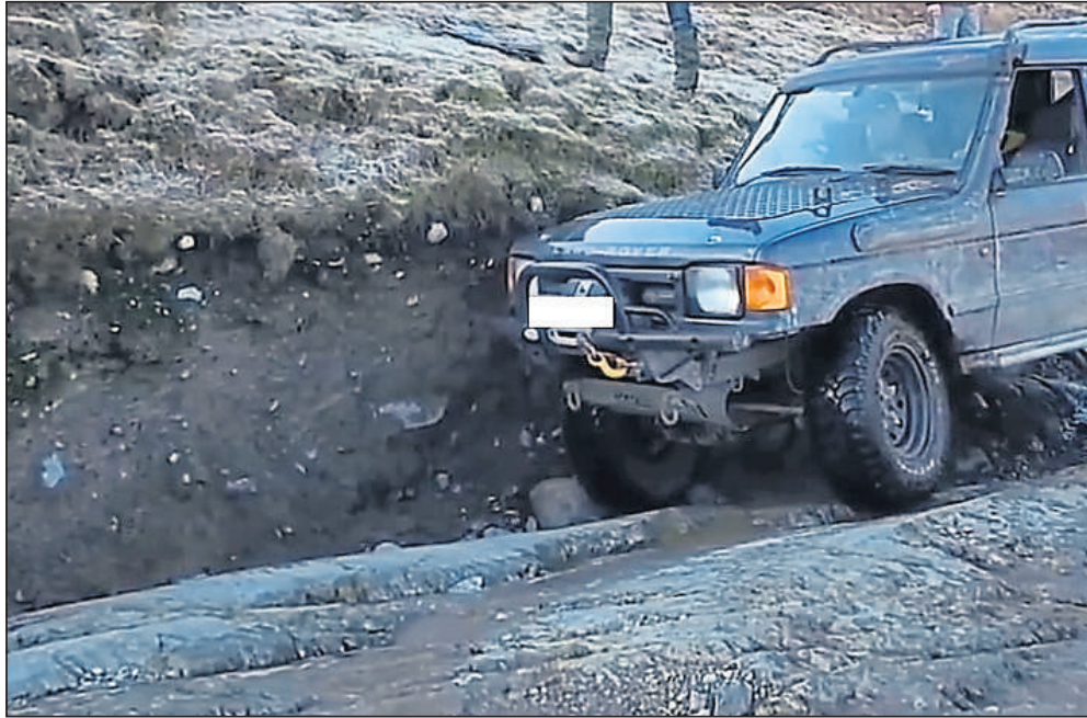
Damage to the unsealed road which runs through Tilberthwaite Farm
