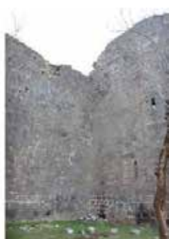
Fig. 26, 27: 19th Tower: New stone falls were noted on the northwest façade's upper corner. Cracks have formed, and the danger remains. There are also new stone falls at the tower's junction with the wall to the north.
