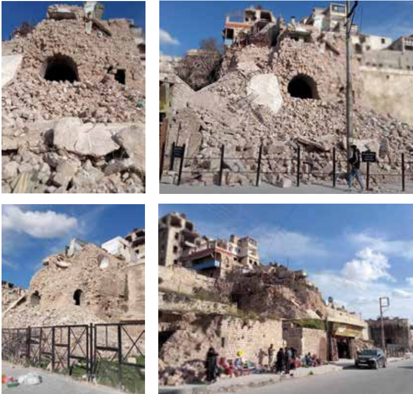
Fig. 1–4: Almost complete collapse of a tower on the western wall of the city, the earths devastation.
