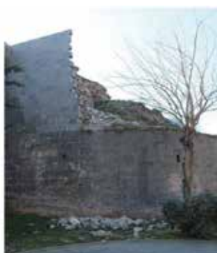
Fig. 51: 11.02.2023 79th Tower: The earthquake caused stone ruptures and falls from the inner fill on the eastern façade.
