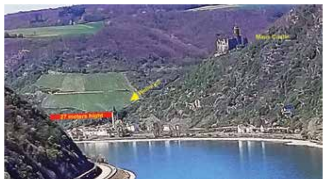
Fig. 14: The bridge, which according to the expert opinions is 27 m high and 450 m long, is almost as high as the belfry in Wellmich. The landscape will be dominated by the bridge. Photo: Klaus Thomas
