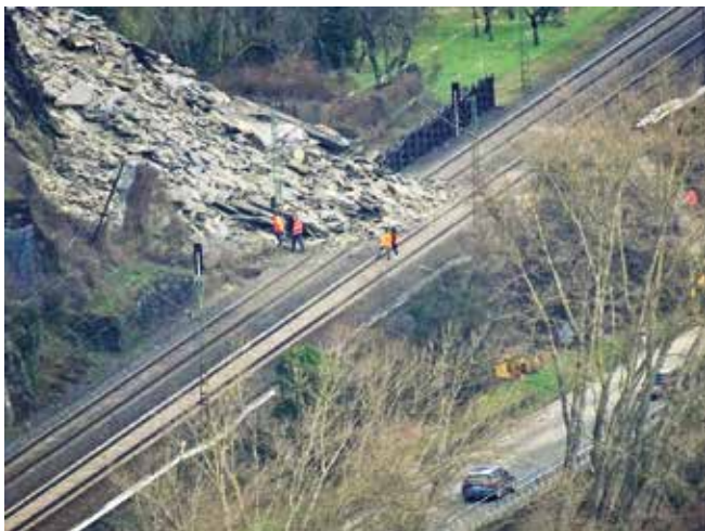
Fig. 17: Landslides on the Rhine are not rare, and extremely dangerous. If trains carrying hazardous goods derail as a result, disaster can occur. Freight trains do not belong in the narrow Rhine Valley. In the short term, however, their speed must be reduced to a maximum of 50 km/h. Photo: Klaus Thomas
