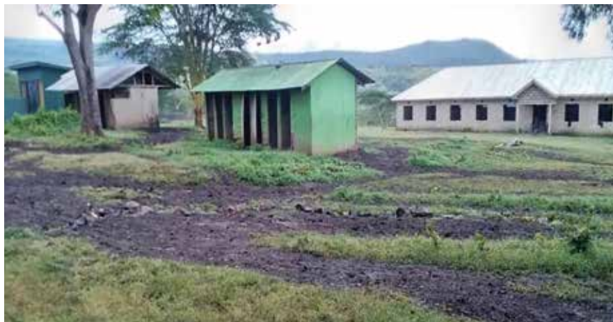
Fig. 4: The school compound in Endulen is deserted, and construction of the dormitory (on the right) has been stopped.
