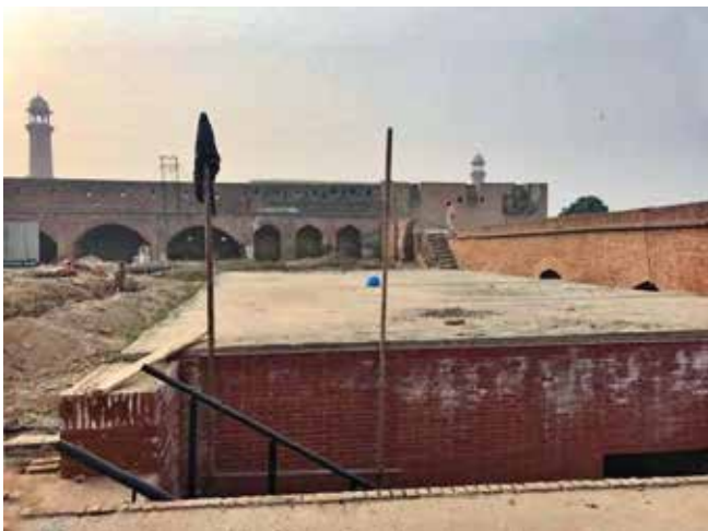
Fig. 3: The roof of the new restaurant showing the extension of the building within the compound of the historic Lahore Fort, 2018.
