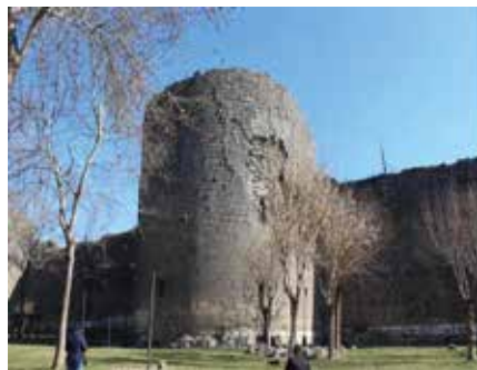
Fig. 23–25: 20th Tower: There are some previously spilled surfaces on the south and north façade of the tower. Several new stone falls have appeared in areas where
