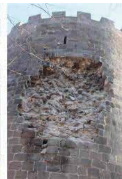
Fig. 47–50: 9th Tower: A large portion of the western façade collapsed. The destroyed area and its surroundings bear risks. There is also swelling on the northern façade and a high level of humidity.
