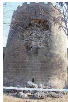
Fig. 47–50: 9th Tower: A large portion of the western façade collapsed. The destroyed area and its surroundings bear risks. There is also swelling on the northern façade and a high level of humidity.
