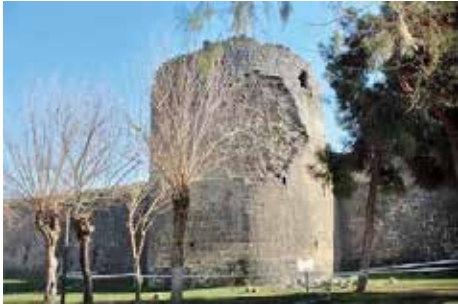
Fig. 42–44: 16th tower: On the surface, there are new collapses and swells. It bears risks in previously destroyed areas on the northern façade.
