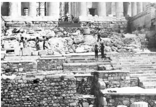
Fig. 7: View of the west access of the Acropolis from the west, about 1980. The restored steps from the 1850s are missing, because they were considered too intrusive. They have been replaced by a zig-zag ramp in a lower level, following the plan restored by Gorham P. Stevens (see below, fig. 8), which most probably was in use for centuries, after the erection of the Propylaea. Photo: Tasos Tanoulas
