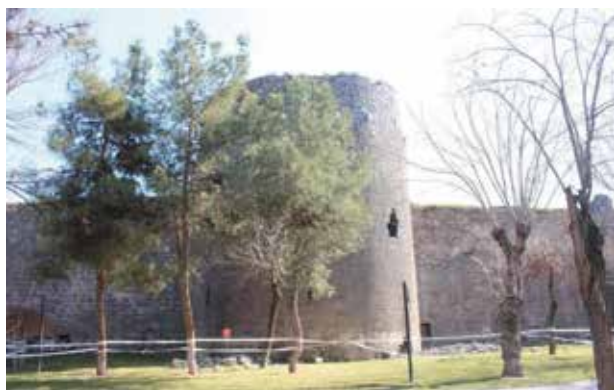
Fig. 30–34: 18th Tower: New stone falls have caused damage to the upper portion of the tower's south façade. Again, as a result of new stone falls caused by the earthquake, the damage in the previously ruined area in the upper part of the western façade grew. A small mass in the upper north façade above the previously devastated surface poses a danger.
