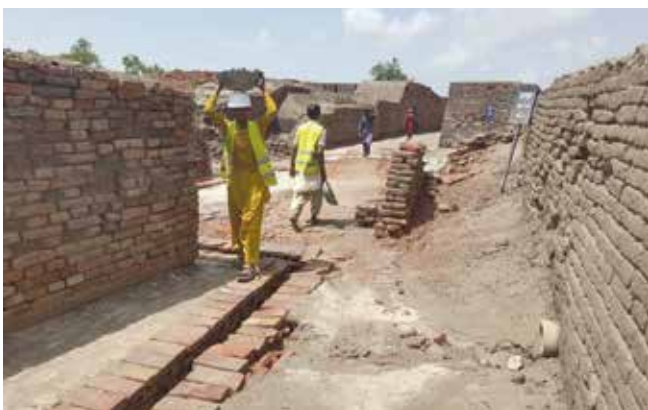
Fig. 3: Conservation works after the floods.
