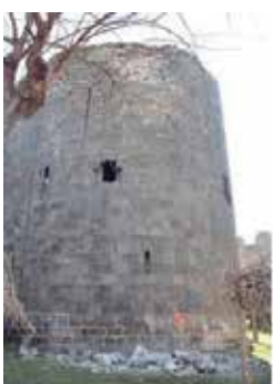
Fig. 23–25: 20th Tower: There are some previously spilled surfaces on the south and north façade of the tower. Several new stone falls have appeared in areas where
