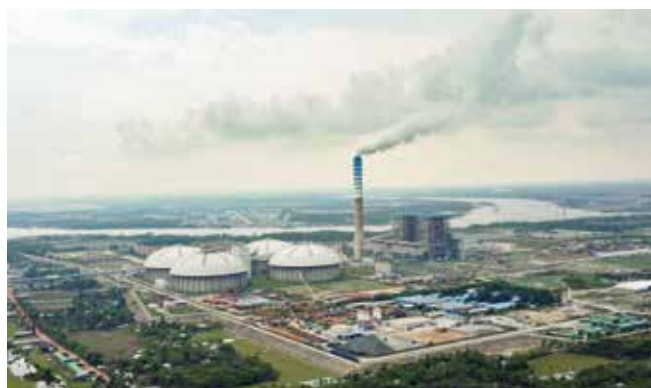
Fig. 2: Drone Photo of Patuakhali Power Plant in Payra.
