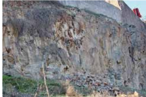
Fig. 55, 56: Rock Layer under the Eastern Walls of the inner citadel: The earthquake destroyed the rock layer beneath the Museum Excavation Exhibition Building. The same rocky surface has numerous cracks.
