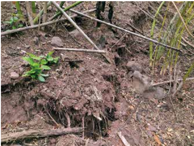
Fig. 7: A crack in this bamboo-covered steep slope hints at an impending landslide.
