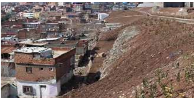
Fig. 9, 10: Rocky Area below Tower 36 and 35: It was observed that large pieces of rock fell from the rock layer at the base of towers 36-35.
