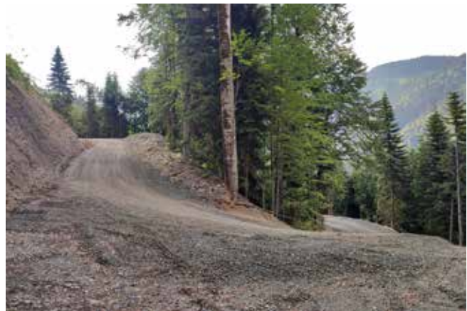
Fig.2: The road in the Sochi National Park (July 2022).
