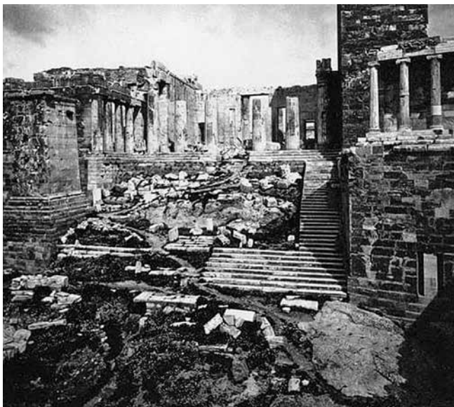
Fig. 6: View of the west access of the Acropolis from the west, after clearing of medieval and Turkish structures. Few of the Roman steps survive in situ. Next to the left wall of the Athena Nike bastion, a narrow flight of steps was reconstructed in the 1850s, after the model of the Roman steps, for providing visitors' access to the Propylaea. Photo: Stillman, 1869
