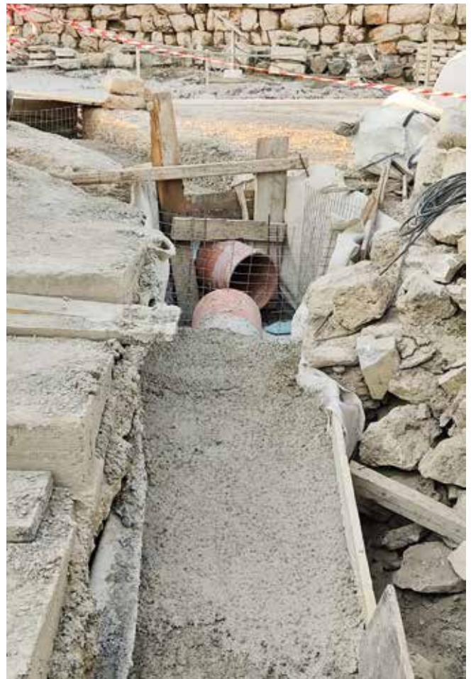
Fig. 13: Part of the rain-water drainage system on the Athenian Acropolis, to the west of the Erechtheion, looking south. From top to bottom: the Parthenon, the foundation of the Old Temple of Athena, channels constructed in reinforced concrete for the accommodation of big plastic pipes (summer 2021). Photo: Tasos Tanoulas
