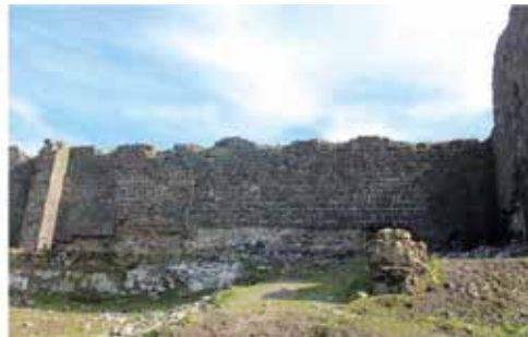
Fig. 13, 14: The Wall between 29th and 28th Towers: It was observed that there were new stone spills in the previously destroyed areas with the earthquake.
