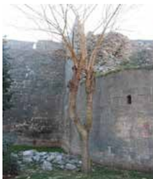
Fig. 51: 11.02.2023 79th Tower: The earthquake caused stone ruptures and falls from the inner fill on the eastern façade.
