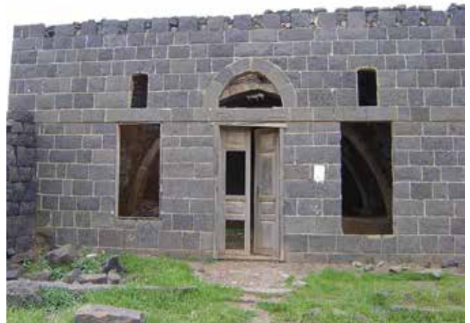
Fig. 8: Façade of a house in Sha'arah. Photo: Y. G. MAFSS
