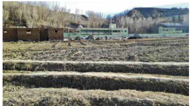
Fig. 3–6.: These pictures show new constructions in the Bamiyan Valley. Photos: Anonymous
