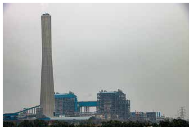
Fig. 3: Rampal Power Plant in operation from Pashur River.
