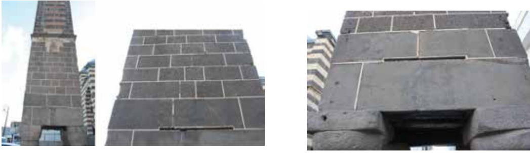
Fig. 62, 63: Four-Legged Minaret: There is a previously existing vertical crack in the middle of the north façade monolithic beam. New separations have also occurred in the joints extending upwards on the beam.
