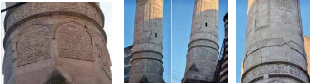
Fig. 62, 63: Four-Legged Minaret: There is a previously existing vertical crack in the middle of the north façade monolithic beam. New separations have also occurred in the joints extending upwards on the beam.
