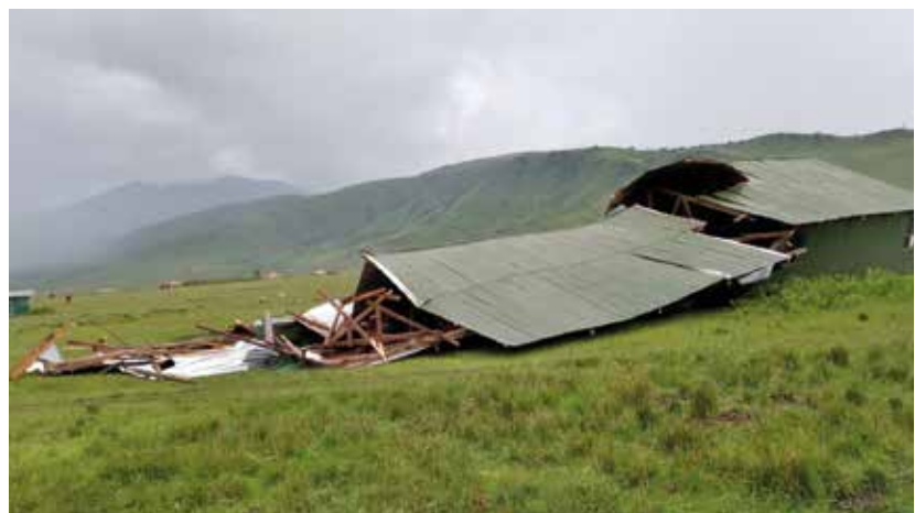
Fig. 3: A house in Oloirobi destroyed by the authorities. Its owner is not allowed to repair it. Photo: Marko Kipuyo
