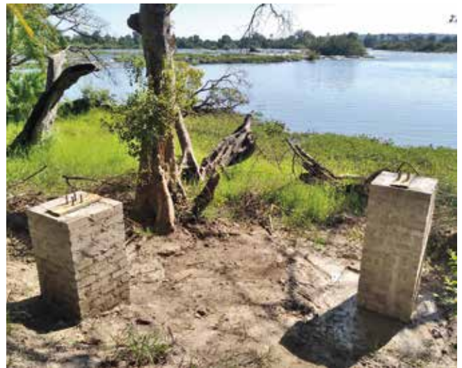
Fig. 2: Riverside Restaurant construction, October 2022. Photo: Keep Victoria Falls Wild
