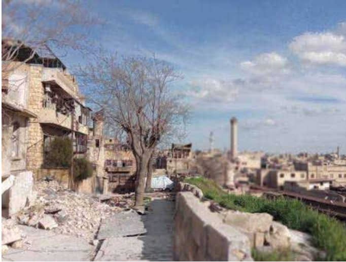
Fig. 10: A general view showing the demolition of the upper parts of many minarets.
