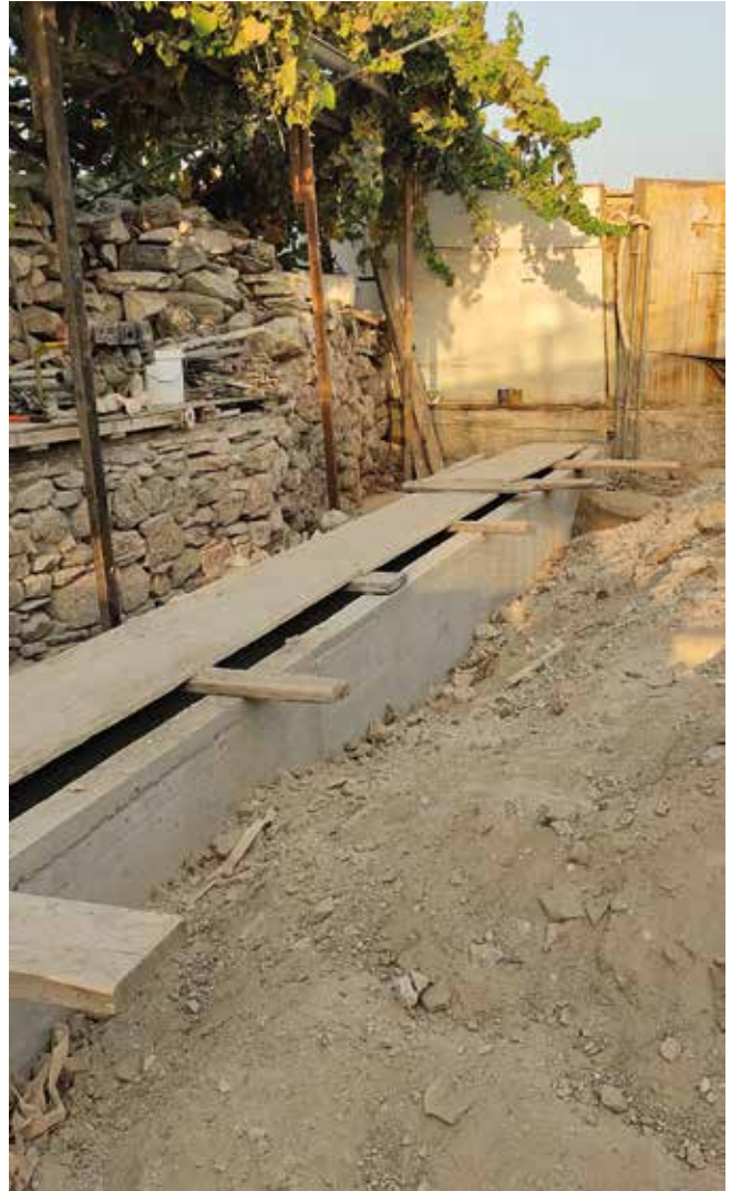
Fig. 16: The same area depicted in Fig. 15, as it was in summer 2021, looking south-west. On the south side, the reinforced concrete channel that was later covered with the metal mesh seen in Fig. 15. The area is not yet filled and paved with reinforced concrete as in Fig. 15 and 17.
