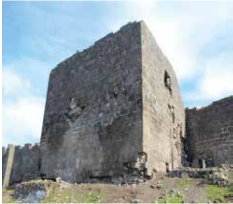
Fig. 12: 29th Tower: There is damage to the surface texture caused by new stone spills, and the risk of stone falling continues.
