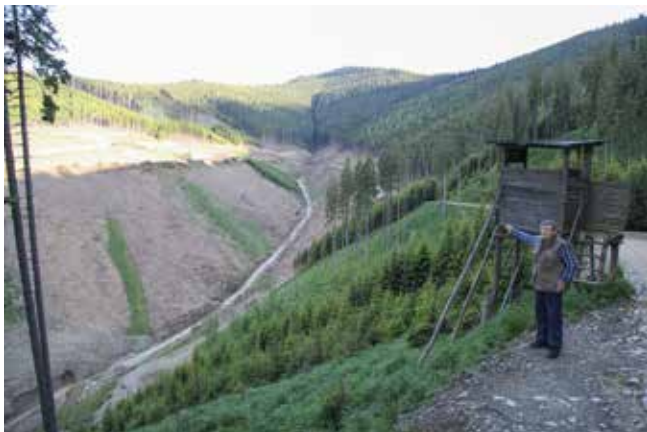
Fig. 4: For the dumping of the SBT excavated material, the forest in Longsgraben was cut down.
