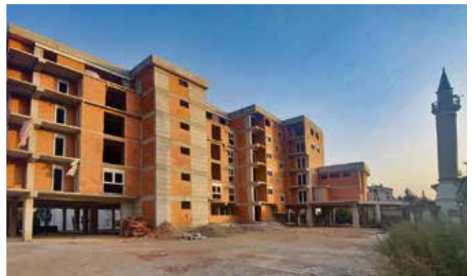
Fig. 6: An apartment block looming over 3 cultural monuments at the Voska Hammam on 19 August 2022 shows a massive advance in construction since early 2021.
