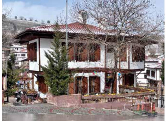
Fig. 4: Reinforced concrete replica hotel in Çukur, Safranbolu. Carelessness reveals itself by the fact that the protruding buttresses are too thin to be a carrier. Photo: İbrahim Canbulat
