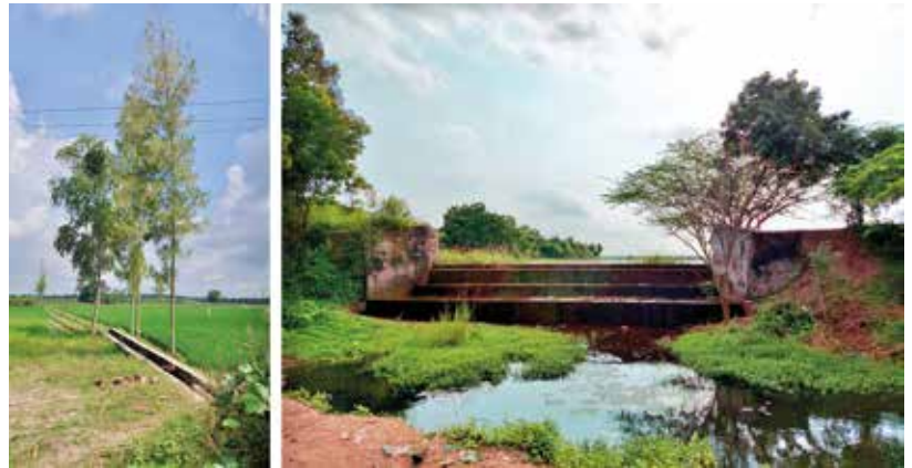
Fig. 6: (Left) Irrigation channel that supplies water to the agricultural fields; (Right) Surplus weir that allows excess water from an eri to reach the next one in a series. Photos: Aghash Natarajan
