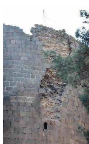
Fig. 38–41: 17th Tower: The shedding of surface stones on the southwest and northwest façades of the tower has resulted in demolition and weathering. It's perilous.
